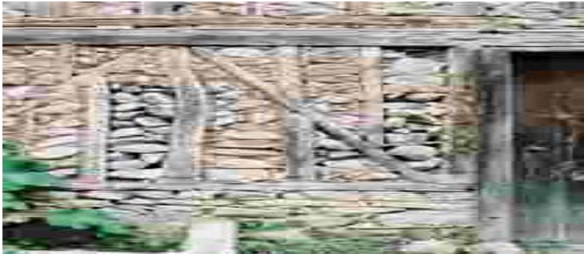
Fig:2. 'DHAJJI DEWARI' construction in Kashmir
